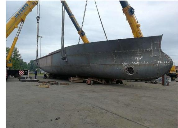
According to the shipyard it is more time, thus cost-efficient, to build the ship keel-up to the main deck and then turn it around with the aid of cranes. This happened 7<sup>th</sup> of September 2021
